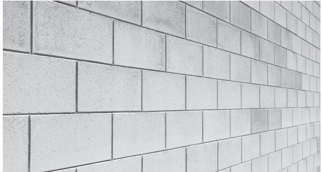
Side view of boundary wall constructed using HCIL Hollow block.
