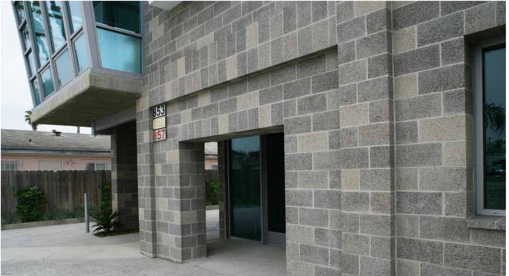
View of how finished construction looks like constructed using HCIL Hollow Blocks.
