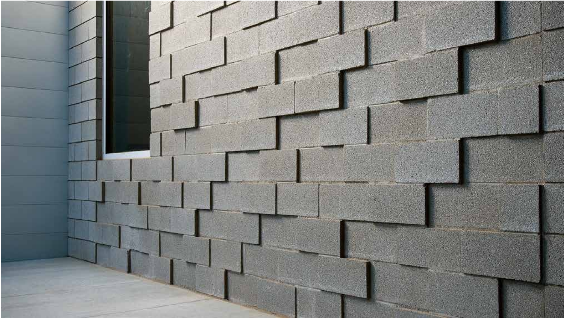
A nice Architectural design constructed using HCIL Hollow Block.
